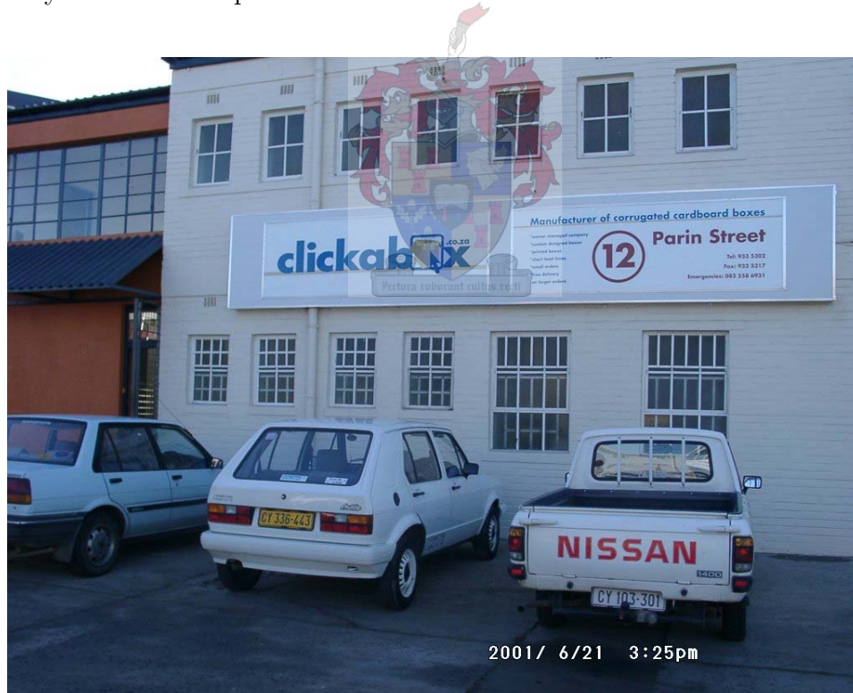
Figure 3.1: View of Clickabox from Parin Street . The office block and parking lot are visible. To the left of the (white) office block the receiving goods entrance is visible, whilst the finished goods exit is just off the photograph, to the right.
